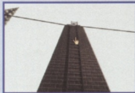
The Power line, prone to circuit breaks.
